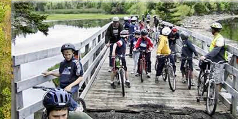
Deepdale Trestle 111.6 m long, 24.4 m high
