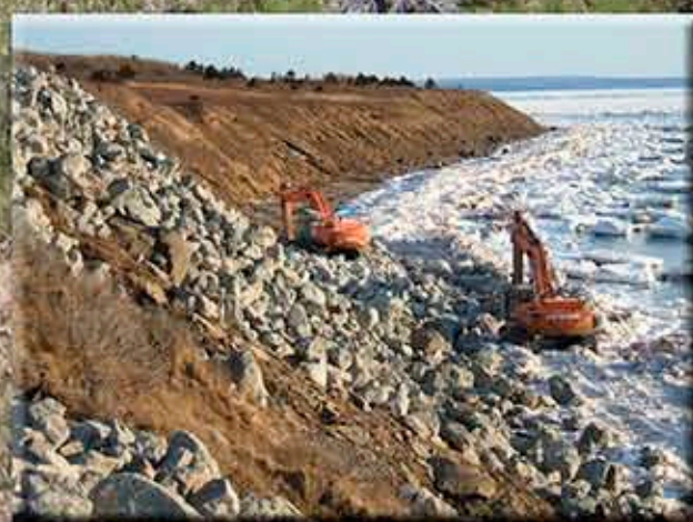
In March 2008, over 1100 trailer loads totalling 23,000 tonnes of armour stone was placed to protect the trail from coastal erosion and storm surges.
