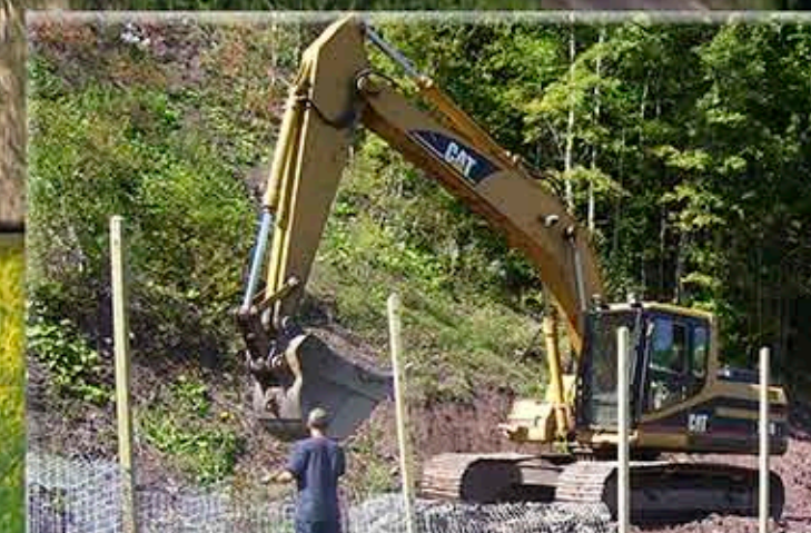
Gabion wall installation at Glendyer.
