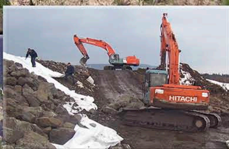
In March 2008, over 1100 trailer loads totalling 23,000 tonnes of armour stone was placed to protect the trail from coastal erosion and storm surges.
