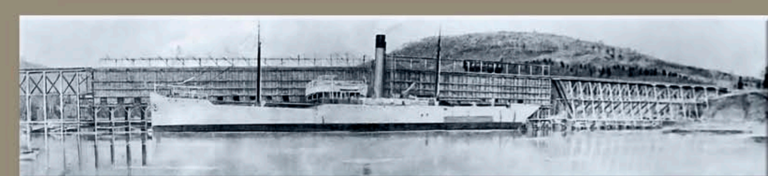
Shipping Pier & Trestle N.E. Mabou 1905-06
