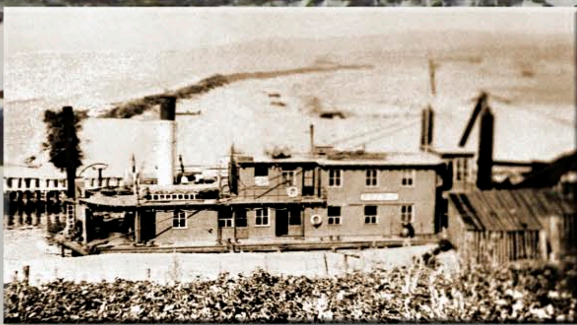
Dredging, circa 1922 This was an ongoing activity due to build-up of sand in the narrow opening.
