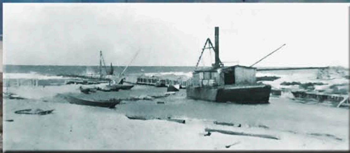
Dredging Broad Cove Coal Mines channel, circa 1894
