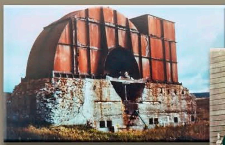
Fan House (out of service), circa 1958
