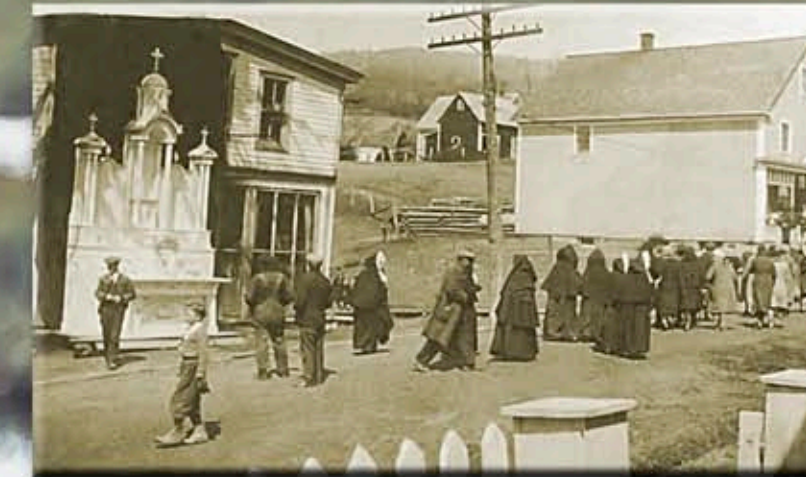
Altar built and guided by Tom Burke, master carpenter, circa 1920 Mabou. The building at right is the current An Drochaid museum.
